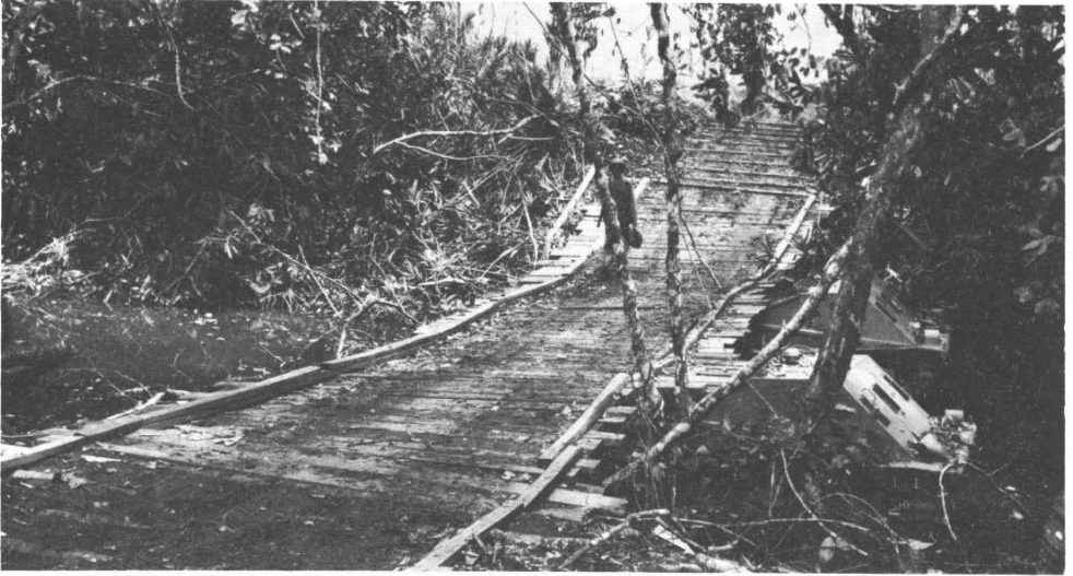
MARINE ENGINEERS erected this bridge across the Tenaru River to speed the flow of troops and supplies from the beaches to the perimeter. (USMC 50468-A)
